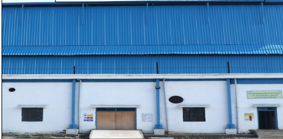
Fly ash based LWA Facility
