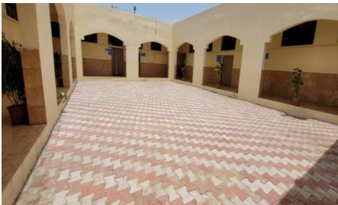
12000 Interlocking paver blocks used in Sipat
